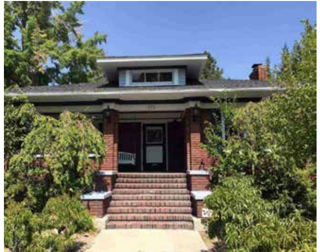
The owners of 571 Ridge Street (built in 1931) received a grant in 2017 for a variety of projects including contractor site work, carpentry and stucco work, painting, and gutter replacement.
